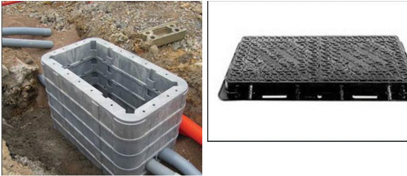
Plate 4.11 Fibre Chambers (construction and external appearance)
