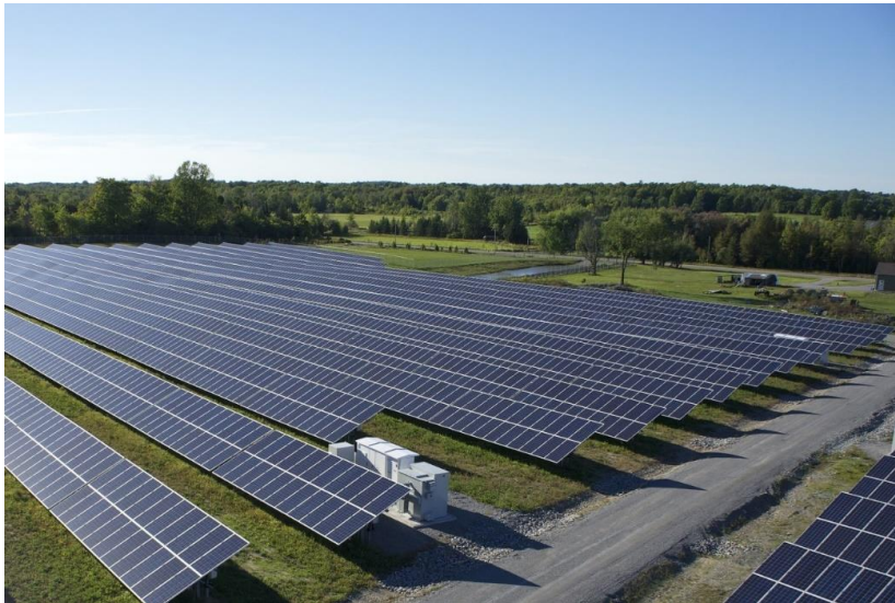
Plate 4.2 Typical Fixed Panels (with Inverters)
