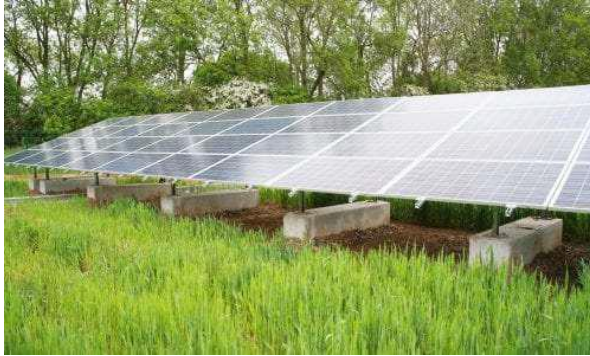
Plate 4.3 Panels on Concrete Feet
